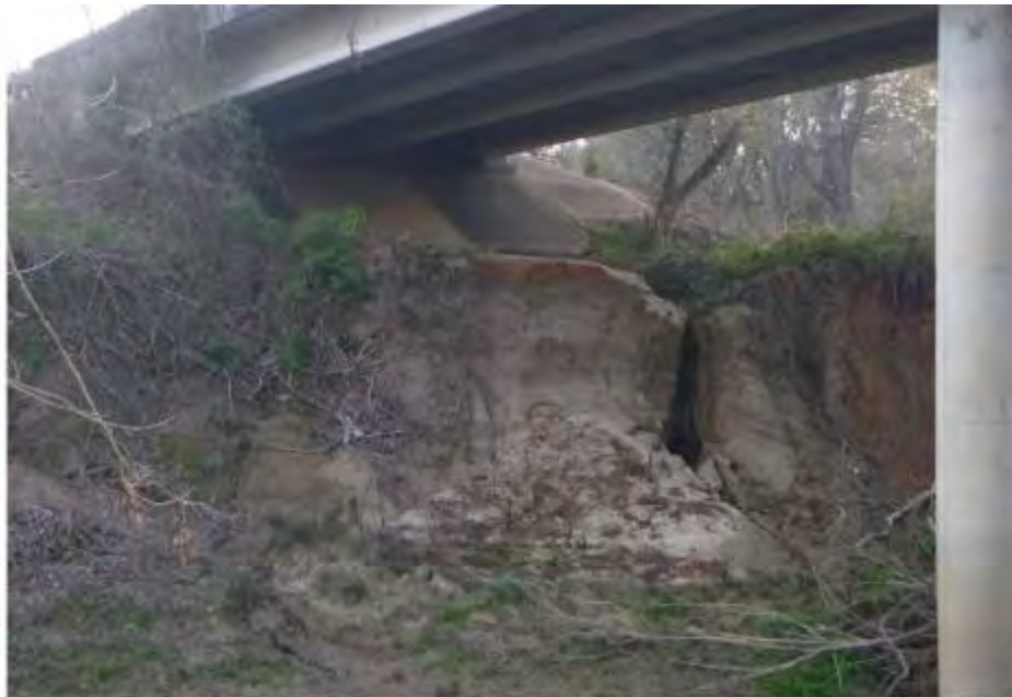
Figure 46. Local scour erosion with 5 feet of bridge pier exposed, 2020. Photo by TxDOT.
