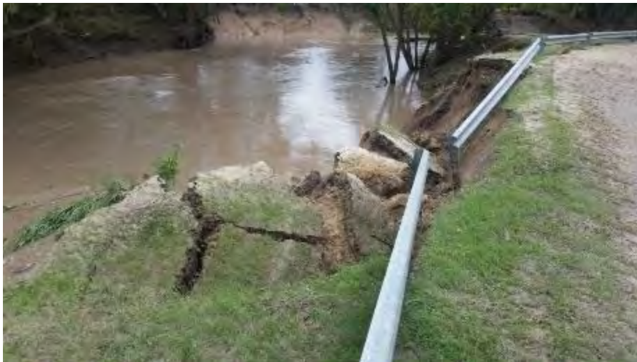
Figure 42. Road surface damage from streambank erosion, Faunt Le Roy Park, 2019. Photo by kxxv.com.
