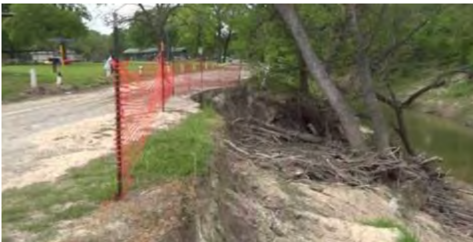
Figure 42. Road surface damage from streambank erosion, Faunt Le Roy Park, 2019. Photo by kxxv.com.
