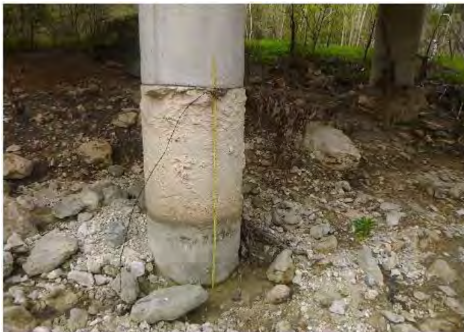
Figure 46. Local scour erosion with 5 feet of bridge pier exposed, 2020. Photo by TxDOT.
